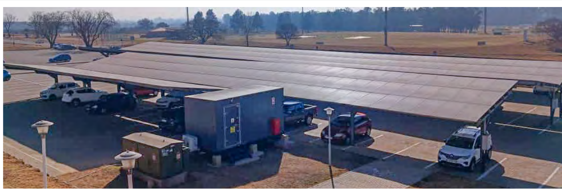
Figure 5: 385 kWp solar panel installed on the carport of the Vanderbijlpark campus (image captured by NWU engineering compliance, 2024)
