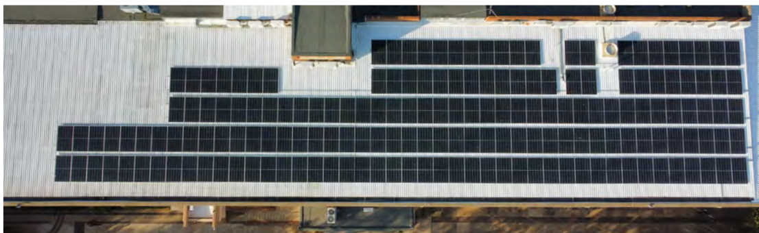
Figure 4: 100 kWp solar panel installed on the Library of the Mahikeng campus (image captured by NWU engineering compliance, 2024)
