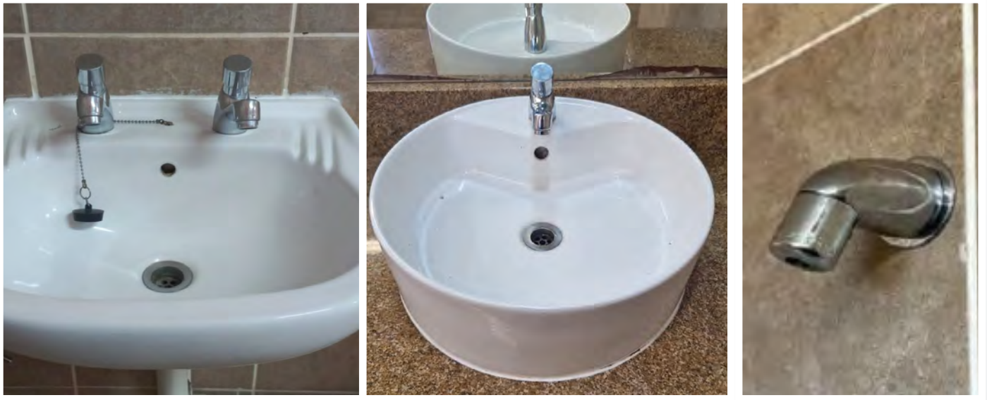
Figure 7: Water saving taps and showerheads installed at residences and office space bathrooms (images taken at NWU residences and office bathrooms)
