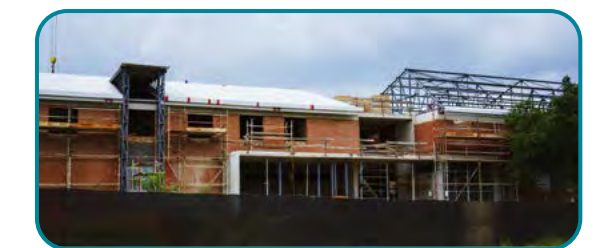
Visible from the road, the new Administration building on the Vanderbijlpark Campus will portray a cutting-edge image for the university.
