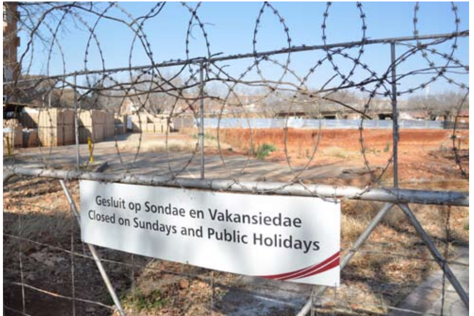
This peculiar notice is on the gate to the building site where the E5 building will soon rise.
